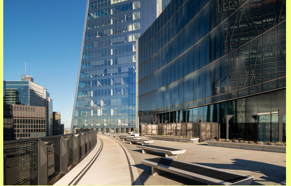
23rd floor terrace
